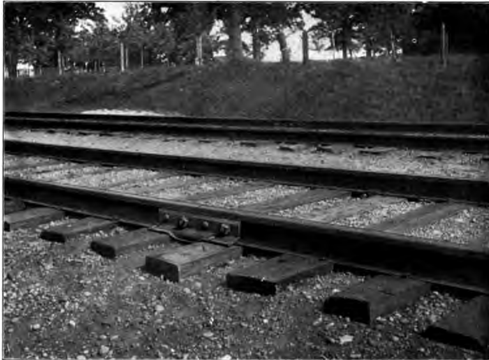
The Railroad, as shown above, has over 3,000 miles of track equipped with 'Bonzano' Joints
